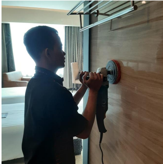
Gambar 10. Polishing bathroom wall
